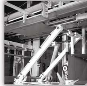
KD case is delivered from elevator to opening station
